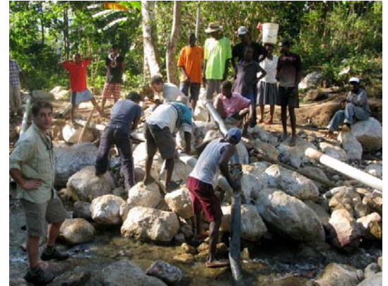
Repairing the distribution system
